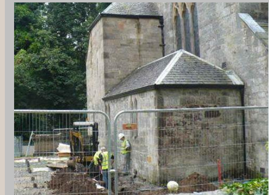
Contract works underway at this church including major groundworks.
